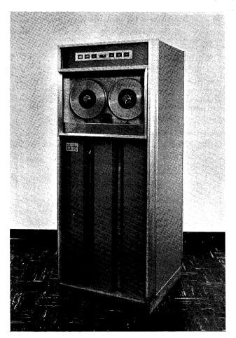
Fig. 1-Type 804 magnetic tape mechanisms.
