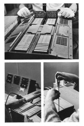
The AN/ASN-24 (G) was designed for exceptionally simple testing, service, and repair. Accurate, uncomplicated test equipment and procedures help to speed check-out and fault isolation. Modular "buildingblock" construction helps to facilitate the replacement of defective units.
