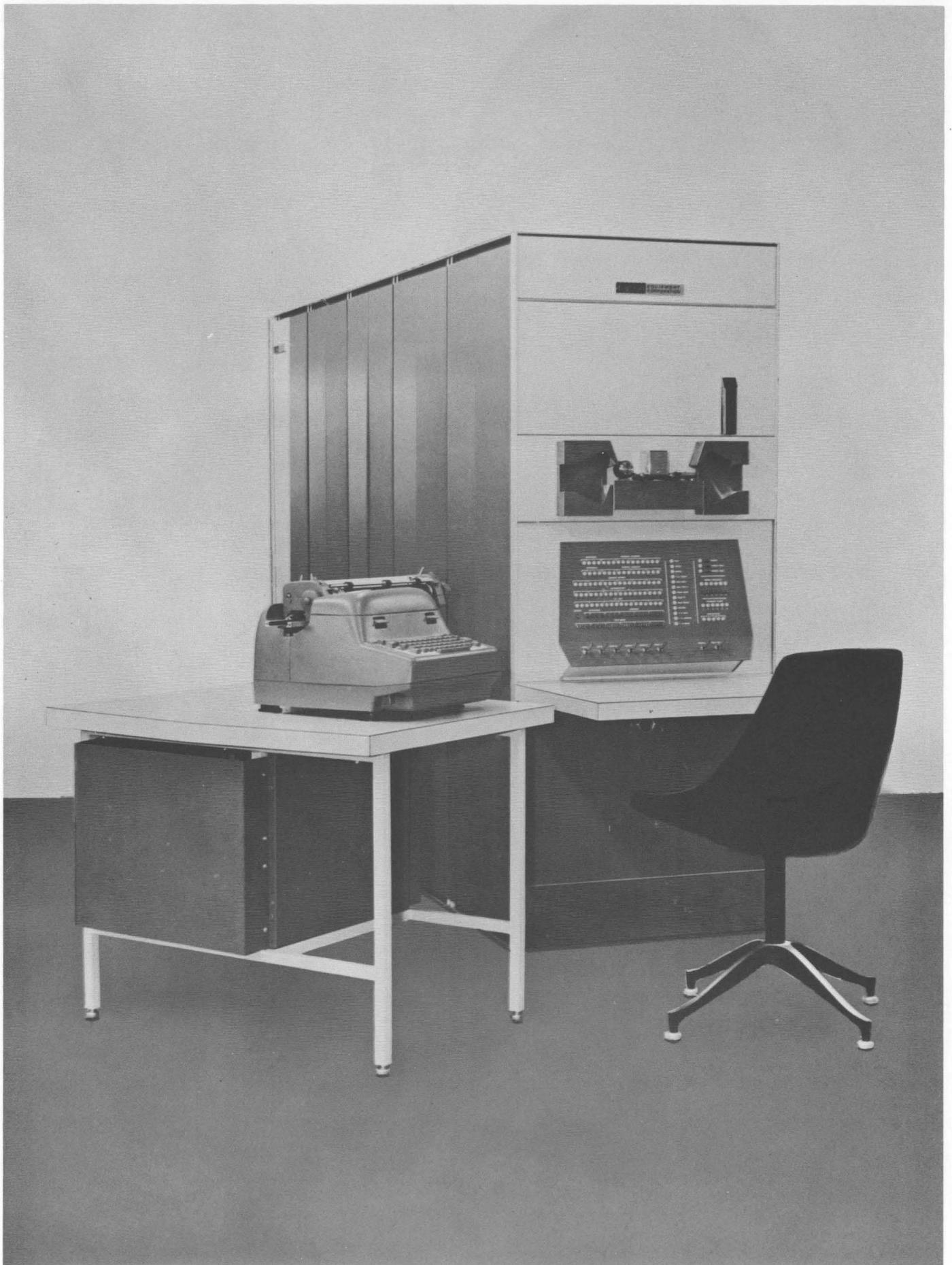
Figure 2-2 Standard PDP-1
