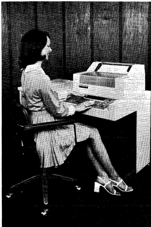
Potter's new diskette data station accepts keyed data and stores the formatted records on a floppy disk, or diskette. These records can be transmitted to either another data station at a different location or to a central IBM computer. A 180-lpm printer produces a formatted hard copy of the keyed data.
