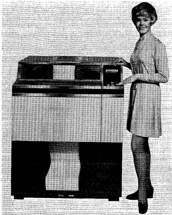
This plug-compatible replacement for the IBM 1403 Model N1 Printer and 2821 Control Unit employs compressed type in order to contract printouts to 10-5/8 by 8-1/2 inches. The Grand Slam operates at a moderately higher speed than the IBM printer while providing the standard IBM features. Both on-line and off-line models are offered.
