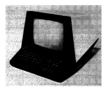
The TEC Model 501 provides a teletypewriter-style keyboard, cursor sensing and addressing, a page or roll-up mode, and switch-selectable transmission rates.
