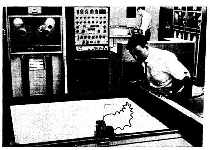
**Dataplotter** in Chicago receives information via telephone circuits from comr in Minneapolis. It can print lines at more than 200 in. a minute.
