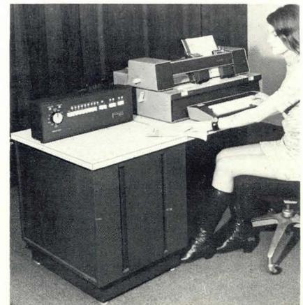
Magnetic Ledger Card Accounting Computer. The Litton/ABS Model 1281 can process letter-sized ledger cards containing 1199 digits per side. Data is maintained on a magnetic stripe positioned at the edge of each card side, with remaining space utilized for account or record printout.
