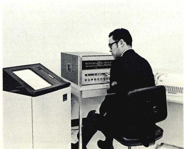
The author of this article, Versatec systems analyst RONALD LEE, is shown here instructing a Hewlett-Packard mini to print-out Teletype-generated data on the Versatec printer/plotter combination at left. In his present position, Lee is responsible for programming and hardware/software interfacing Versatec's complete line of six different hard-copy output devices as well as analyzing customers' system requirements.
