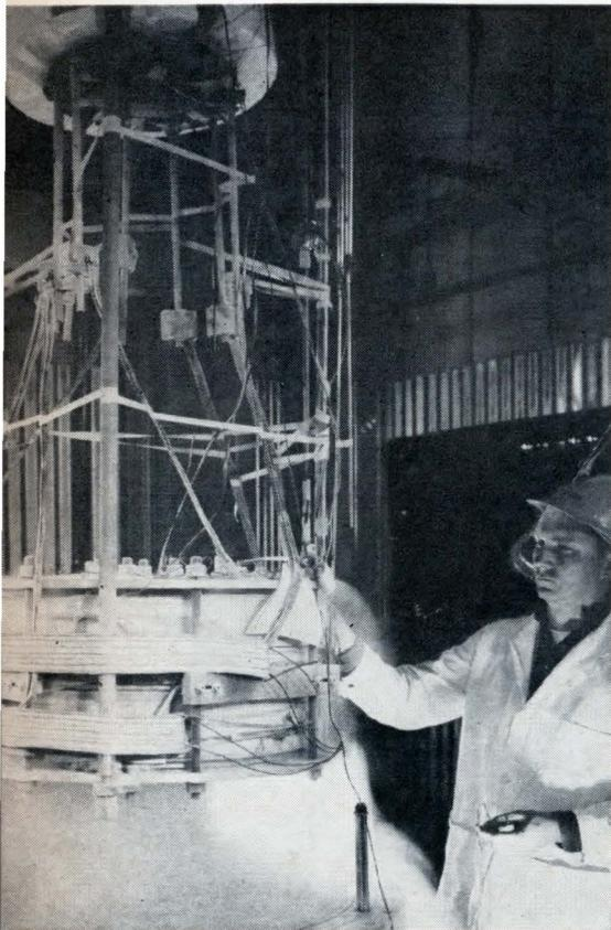
**Wide-bore magnet** provides elbow-room for scientists conducting research on subnuclear particles. This magnet, developed at Argonne National Laboratory, has an 11-inch bore and provides 42,000 gauss.
