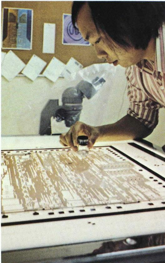
An 80X blowup of the artwork, is made for alignment and circuit verification.
