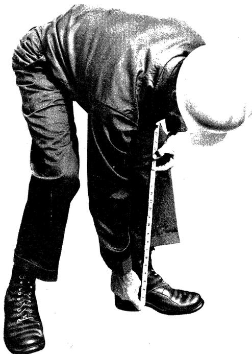
Fig. 8—Measuring for Climber Length
