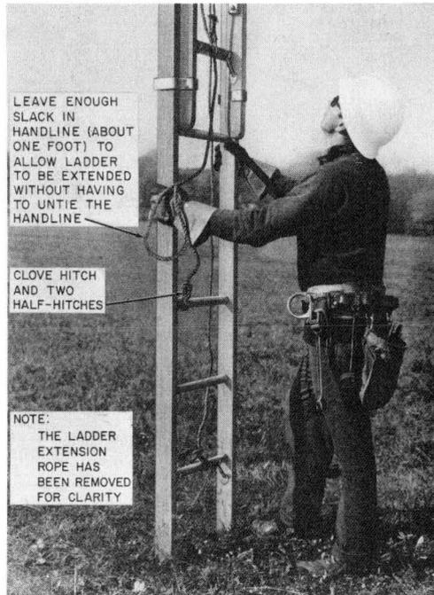
Fig. 20—Method of Securing Handline
