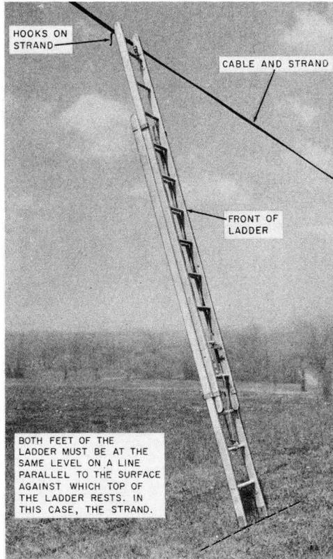
**Fig. 12—Base of Ladder Properly Positioned**
