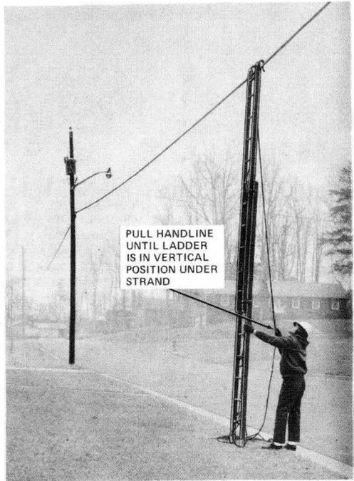
Fig. 19—Ladder in Vertical Position
