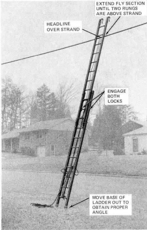
Fig. 21—Ladder in Working Position
